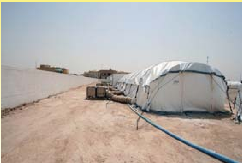
The flysheets and AC system will lower the interior temperature in the tents.
