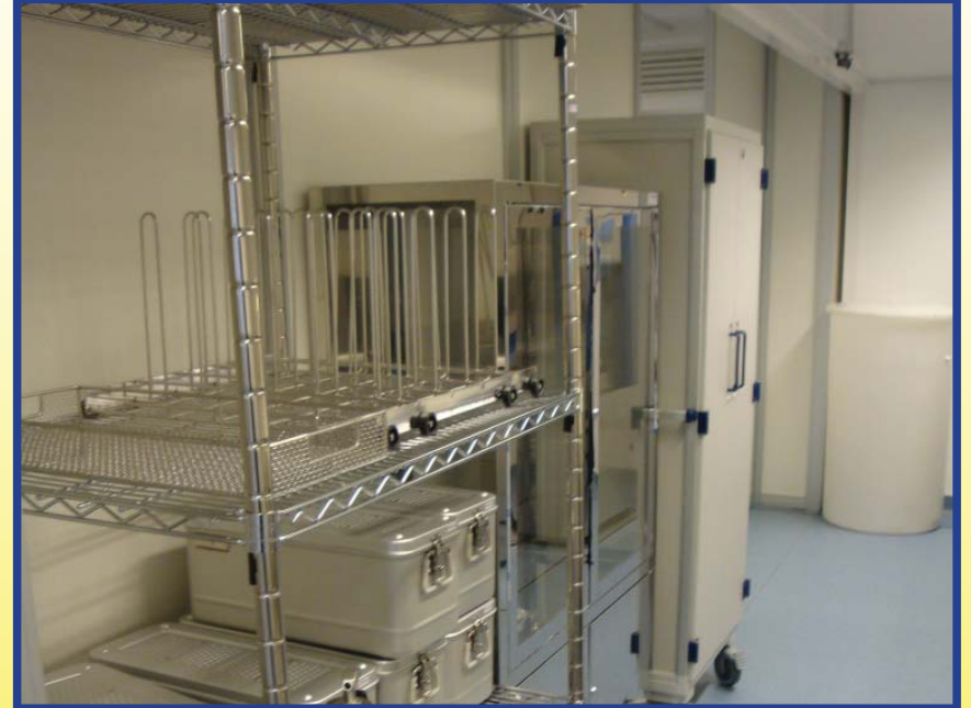
Shelves and environment controlled storage facilities in the sterilization room.
