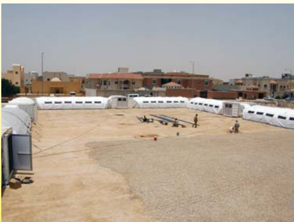
Overview of the hospital area.
